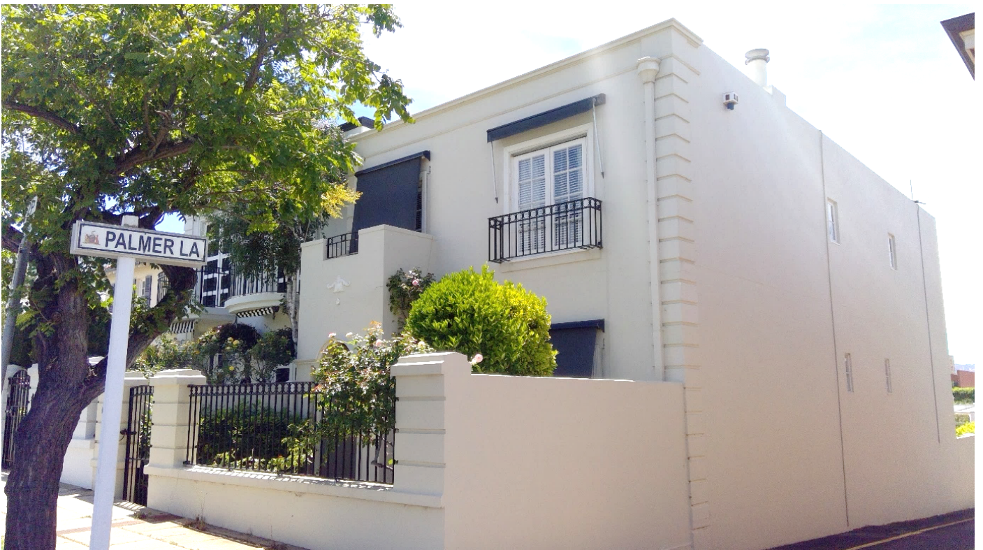
Photo 3.6: View of adjacent dwelling to north at 85 Palmer Place
