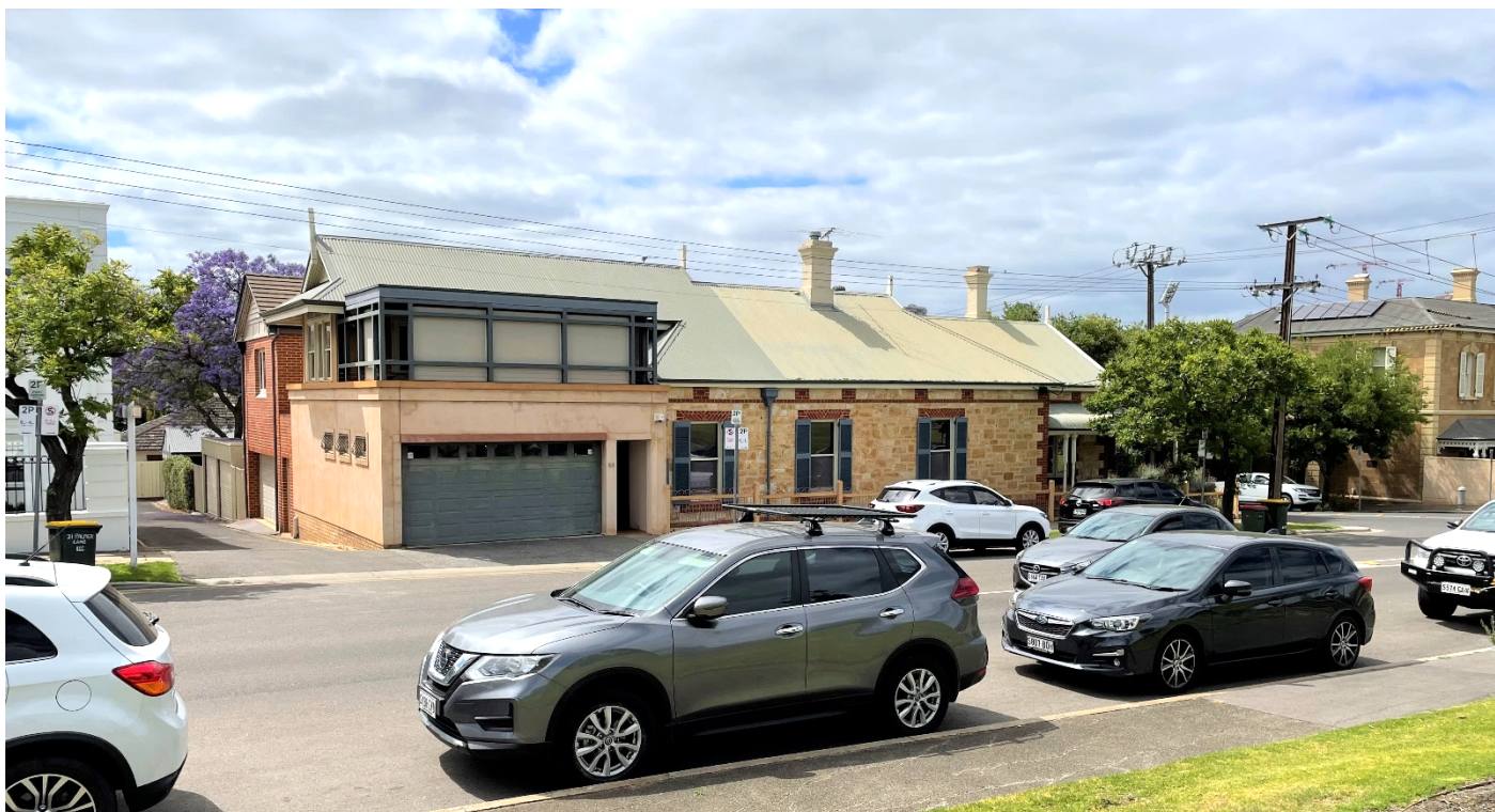
Photo 3.1: View of subject site from Palmer Place
