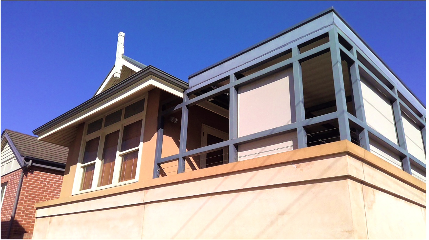
Photo 3.7: View of existing upper addition
